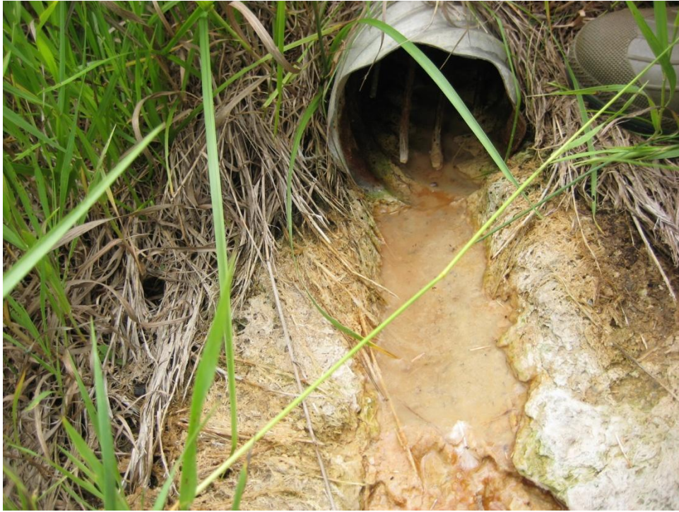
Figure 4.1. Yellowish tufa precipitates at the subdrain outlet
